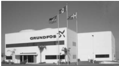
GMX - Monterrey, Mexico
